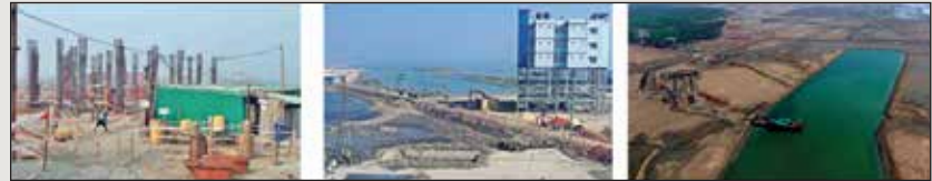
Construction work of Matarbari Power Plant
