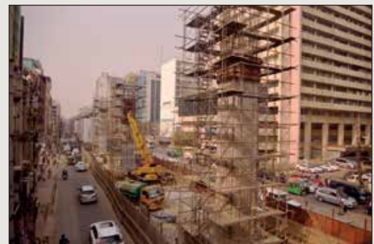
Construction works of MRT-6 in Dhaka city
